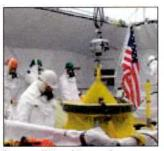
Crews pull the old pump from Tank AP-101, making room for a more powerful pump to feed waste to a treatment plant for glassification.
